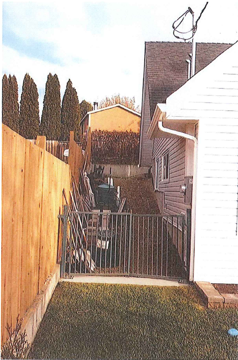
West Side of Accessory Building
